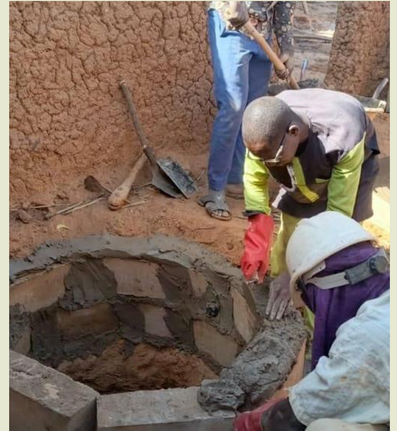
Placing the slab
