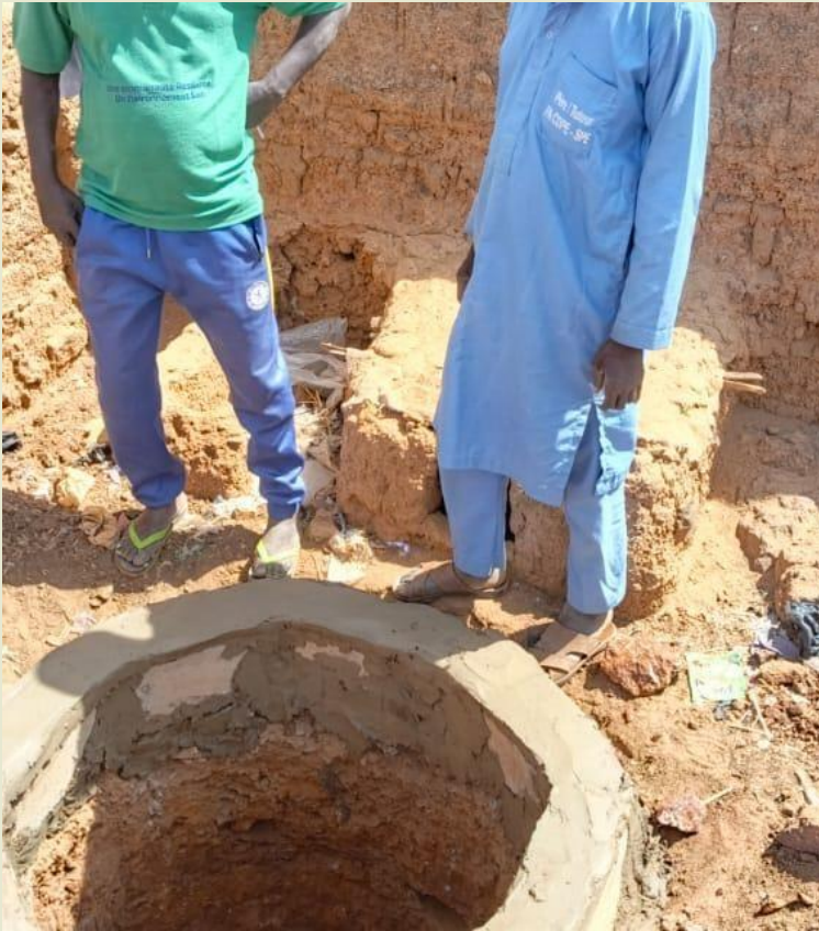
Lining the pit
