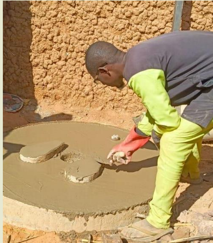
Finishing the slab
